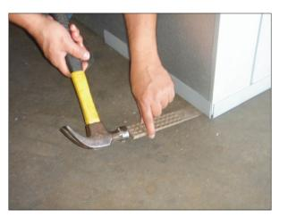
6-Install shims under vinyl screed corners and across as needed to ensure support panel joints and levelness of panel.
