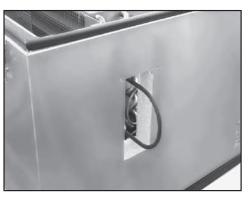
Replaceable heater and access panel
