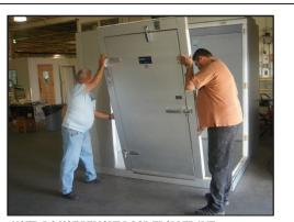
**NOTE: DO NOT REMOVE DOOR FROM FRAME** 7- Door frame must be level with adjacent and flush (on top) with adjacent wall panels. Measure the top and bottom of the door opening to make sure both measurements are the same. (see page 8 for details)
