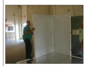
4- Begin with two Corner Panels and secure to Floor panels to start making a corner. <u>Make sure that the top of each</u> wall panel is flush with each other.
